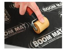
4. Once in the proper location, use your Boom Mat installation roller (050218) and apply pressure to ensure a strong bond between Boom Mat and the installation surface. Design Engineering, Inc. thanks you for your purchase!
